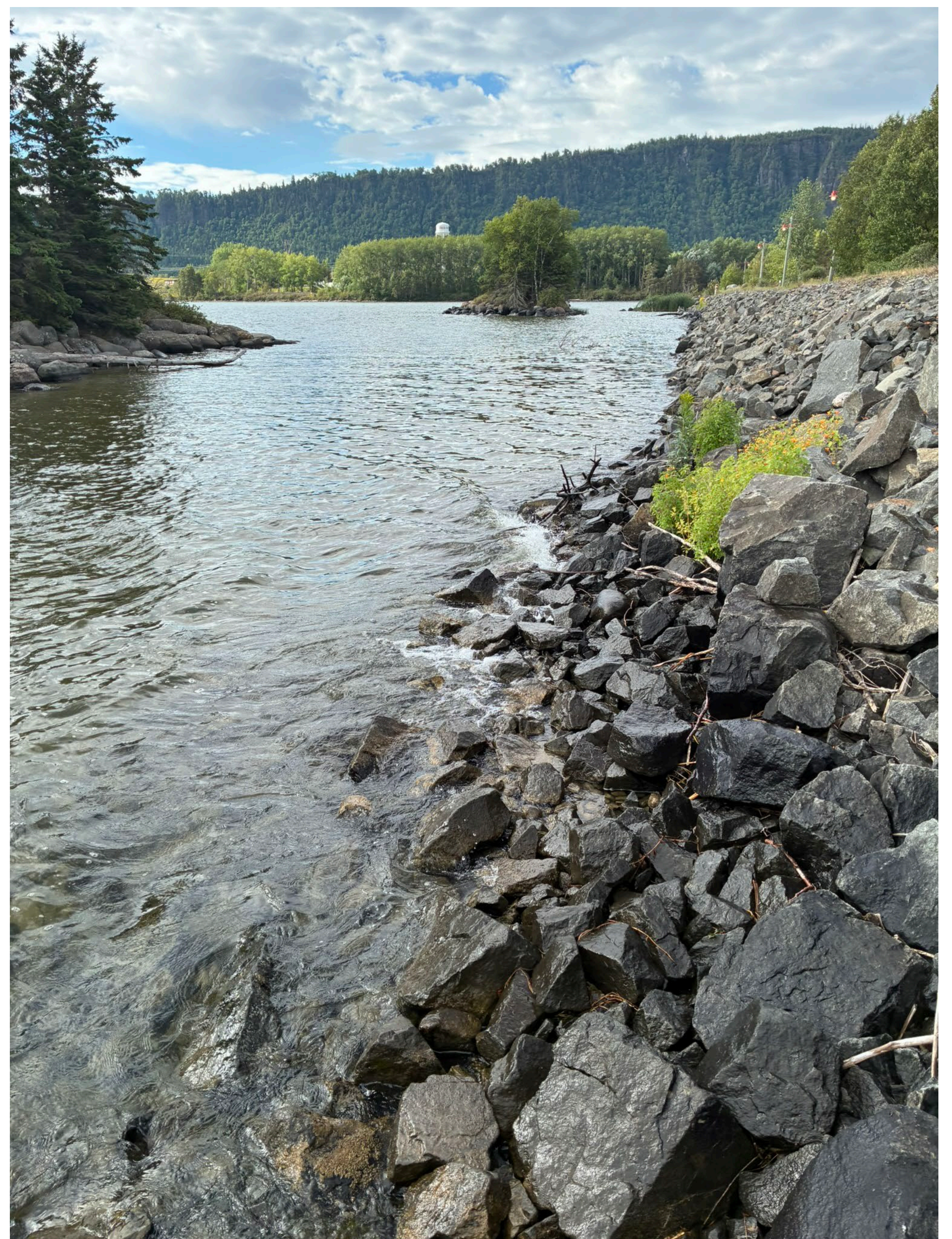
PHOTO - OFF THE BREAKWATER (SEPT. FIELD VISIT)
